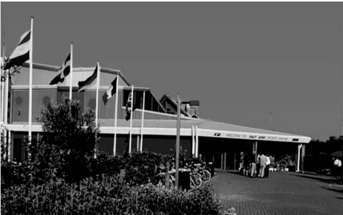
Salt Ayre Sports Centre - the acceptance of an offer from the British Cycling Federation of a project capital grant to develop cycling facilities at Salt Ayre was considered as an item of urgent business
